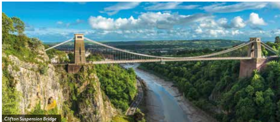
Clifton Suspension Bridge
